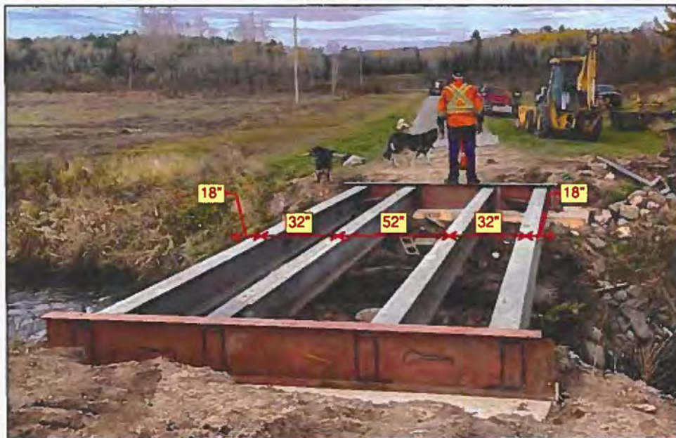
Photograph 1: Overview of Bridge (Under Construction)
