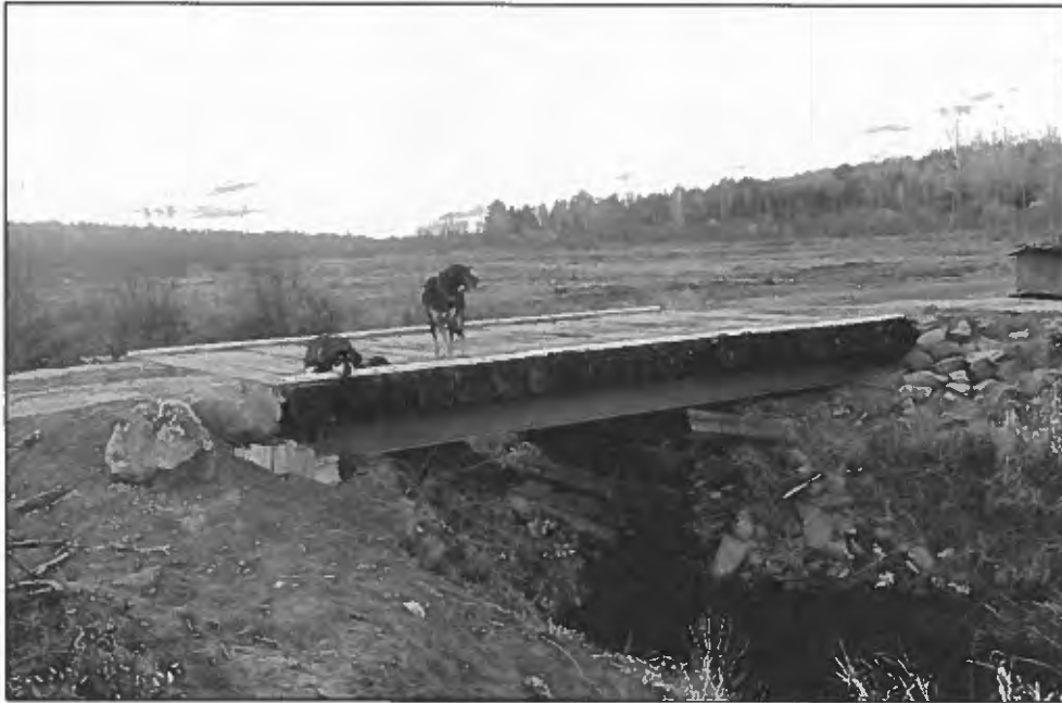
Photograph 2: Overview of Bridge
